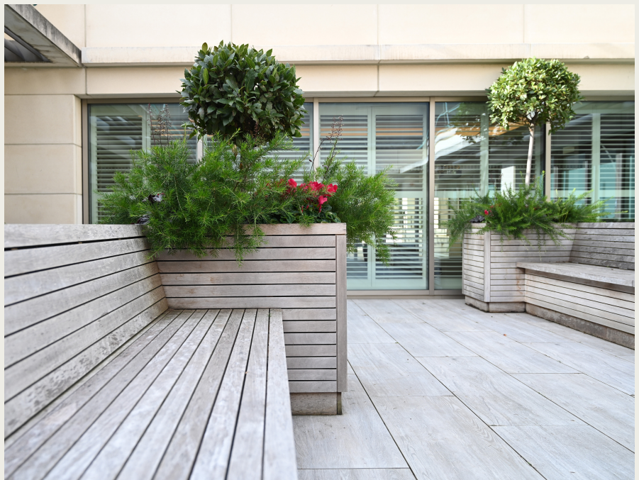
Bespoke benches and planter made from Iroko timber which here has weathered to silver/grey.
